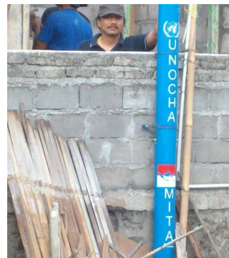
Early Warning system equipment
